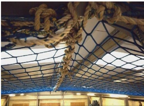
Figure 2. Safety Nets laced together
